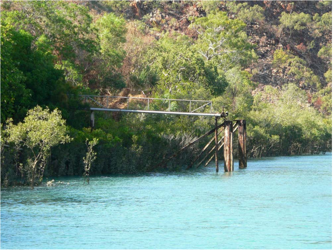
Water pipe at Silver Gull Creek (R Campbell)
