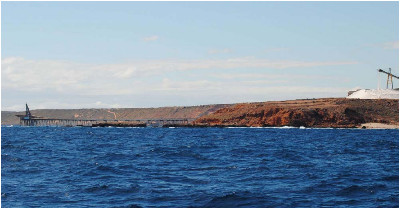
Cape Cuvier salt loading facility - mooring buoys are located other side of the jetty (R&L Newton)
