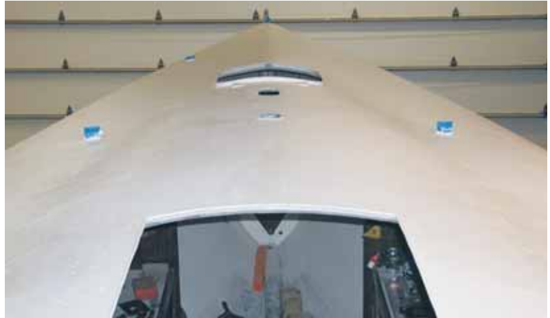
Below—After all this, I was finally back to where I started—ready to start applying new non-skid.
