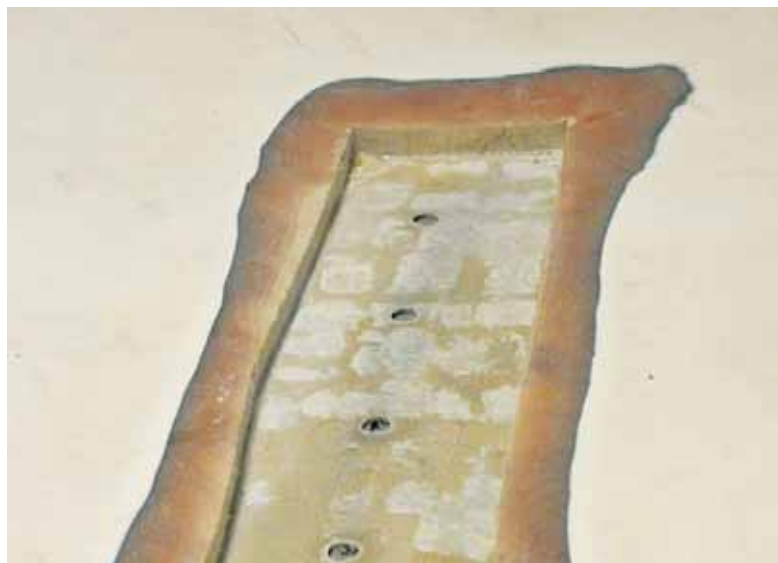
Above —The exposed openings were prepared for repair after the bad core was removed. A 12:1 bevel was sanded into the fiberglass deck skin around the openings.
